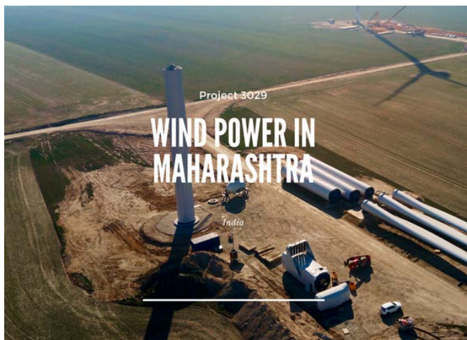
Project 3029: Wind Power in Maharashtra
